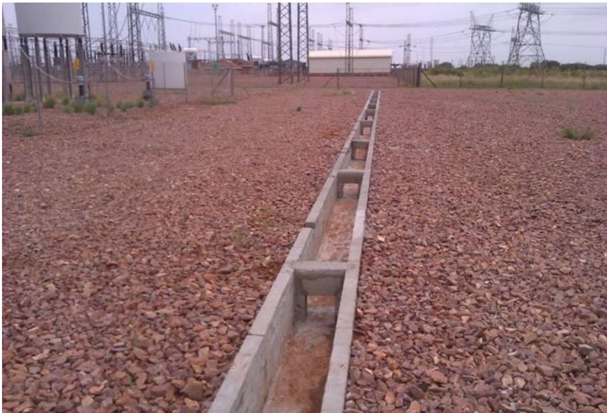
Picture 20 – Drainage ditches with bracing elements (from previous intervention).
